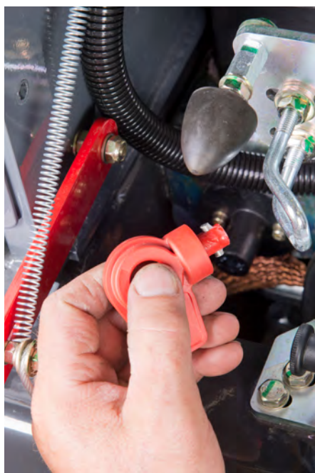
Battery main switch
